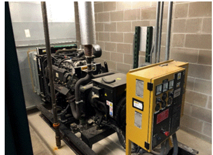
Figure 3: 60kW Generator
