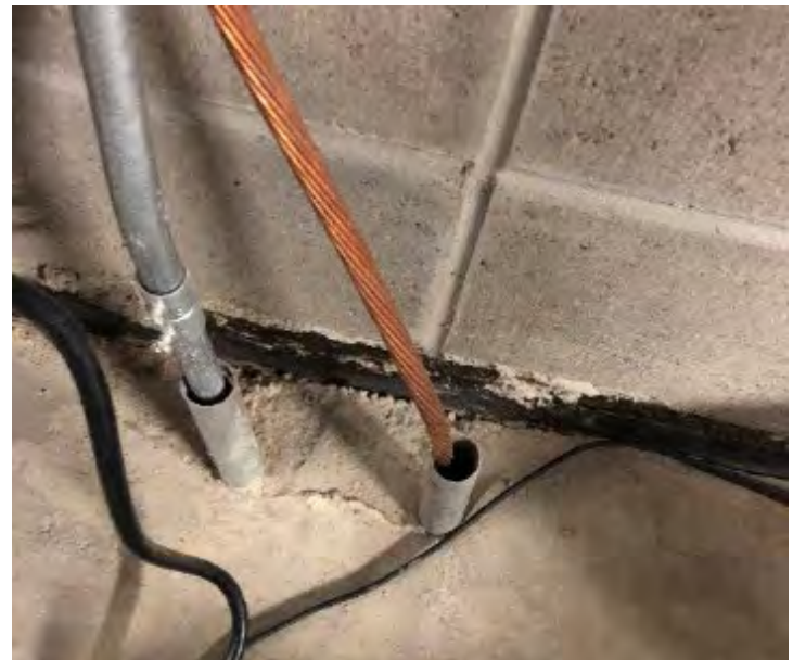
FIG 2: Bare copper ground lead in metal sleeve
