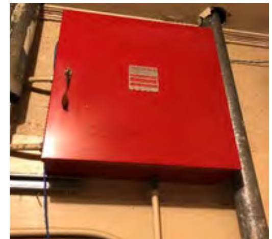
Figure 7: Abandoned-in-place, original fire alarm panel and fire bell
