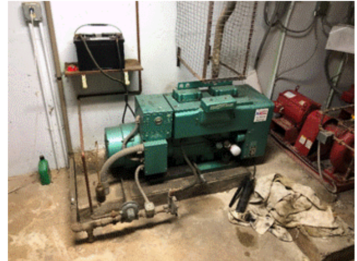
Figure 2: 10kW Generator
