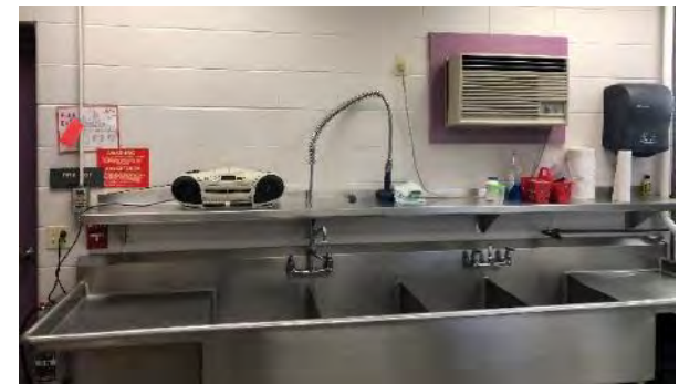
Figure 1: Existing Non-GFCI receptacles installed in proximity of washdown sink
